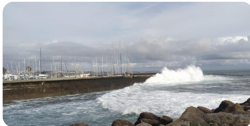
Fig. 3 – The evolution of sea storms caused by climate change impose to reconsider the coastal infrastructures as ports, marinas and other coastal activities. The importance of measure waves variables is crucial for a well-designed infrastructure. (Port of Cascais, Portugal, during a storm event).
